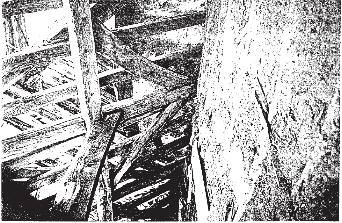
Plate 3: Bracing: north cross wing.
